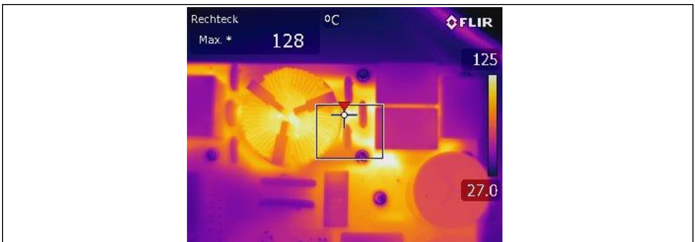
Figure 26 Thermal image of input area
